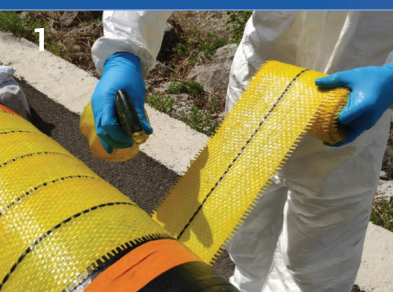
R1D wrapping (spray water continuously)
