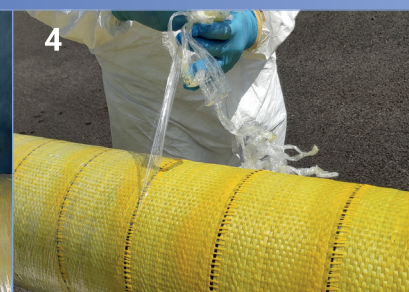
Remove compression film after full curing
