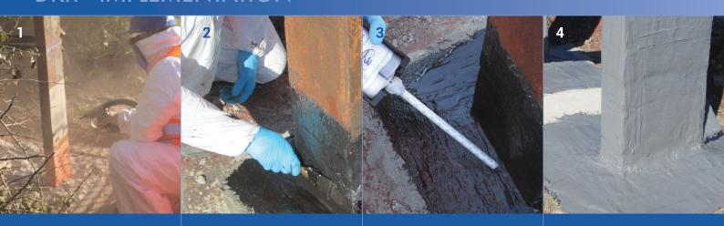
Surface preparation Sa2½ / St3 & roughness Rz > 60 µm (2.4 mil)
